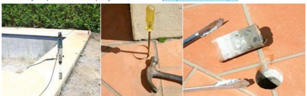
Using a 65mm Core drill, go to a maximum depth of 120mm. remove cores with BBQ tongs being careful not to chip tiles. Remove any debris and dry holes. If going into dirt or garden then dig hole at least 300mm x 300mm x 400mm deep. Fill with quick set or normal concrete and core drill when fully cured.
