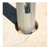
Cement posts into place being careful not to bump posts. Cement should finish 2mm below paving.
