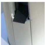
Put the supplied shims on top of your fillets so when you slide the glass into place it sits on top of the shims.
