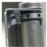
Finally, refit the spring tension pins to the gate hinges and tension so the gate closes from all open positions. Readjust spring tension in 3 to 4 weeks or as required.
