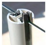
Slide the glass into place. It is best to use two people for this, being careful to keep the glass at as close as possible to 90°. Work slowly. When you have one piece of glass in place, check for height and adjust if necessary {1mmshort of top of post} and then insert two short lengths [20mm] of the glazing rubber at the top of the glass to stop it rattling about
