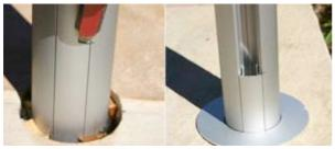
Now measure distance down from top of remaining posts to required point at bottom of posts. On standard fence kits this will be 1170mm which will give you approx 50mm gap at bottom of glass. Remember that the paving can, and most times will be slightly undulating so the overall height will vary. That is why the standard height of the fence is 1220mm and not 1200mm.
