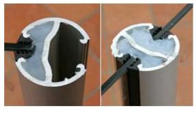
Do one post at a time. Make sure the glass and post is dry before applying the silicon. Apply silicon so that it fills completely the gap behind the glass into the channel, but leave enough room for the glazing rubbers to fit. Apply the silicon and immediately insert the glazing rubbers using plenty of soapy water. If silicon does ooze out, spray soapy water on surrounding surfaces so the silicon cannot spread and remove with plastic spatula or similar device.
