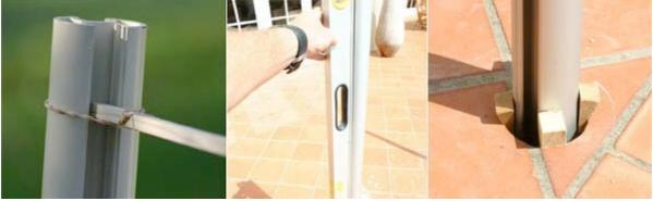
Now using a long level, level post and lock into place using wooden chocks. Do not put chocks in so they cover the glass slot as this is where you will pour in your cement. The spacing sticks will keep the posts at the correct distance apart, you just need to keep the posts in an upright level position. Remember the gate posts will have a different spacer stick!
